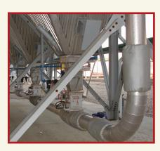
"It was so bad," says Lincolnway Energy maintenance manager, Keith Davis, "that we had to station someone next to the valves to wrap them with a hammer just to keep the material flowing." In the original design for the Lincolnway plant, eductor valves were installed as part of a positive pressure conveying system in the fly ash bag house and the HRSG.
